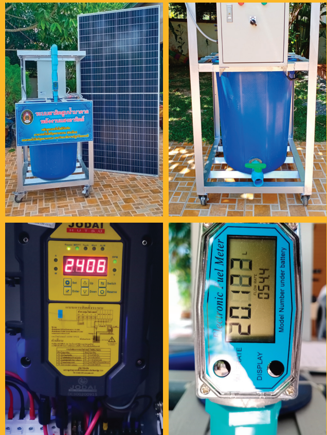
Picture 1: Goal 7 The university is actively engaged in the development of a demonstration system focused on small-scale solar-powered shallow water groundwater pumping for household use. This initiative aims to showcase sustainable and renewable energy solutions by harnessing solar power to facilitate groundwater pumping, particularly for domestic needs. The project seeks to demonstrate the feasibility and practicality of utilizing solar energy for water access in a small-scale, household context.
